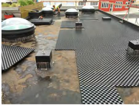
The Atlantis Floccell 20 drainage cell is laid and A19 Geofabric is placed over the drainage cell.
