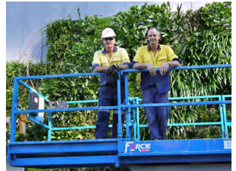
The scissor lift raises the installers and modules to position.
