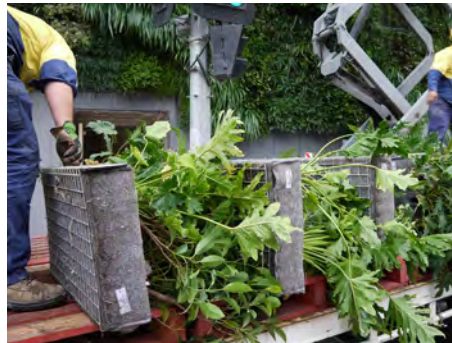
We locate the truck as close to the host wall as possible, unpack the modules directly from the back of the truck to the access equipment.
