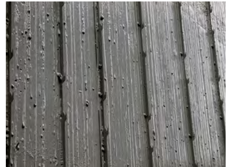
The prepared host wall. We have attached our holding hooks and applied a waterproof protective layer over the entire host wall.
